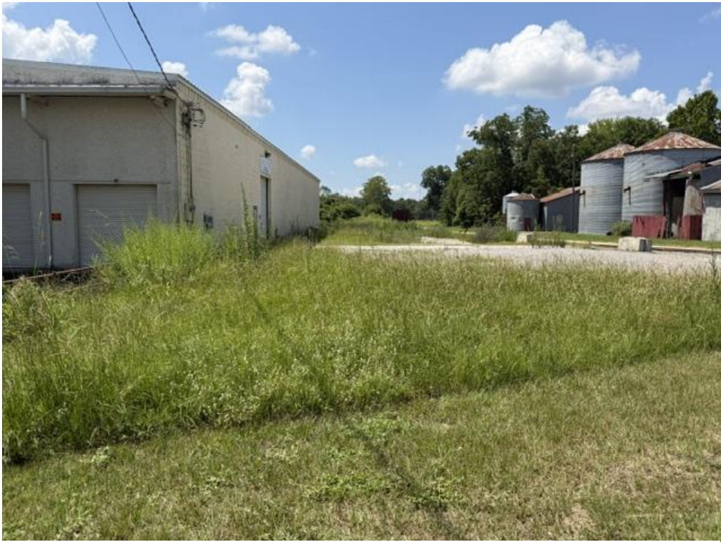
Subject property: view of the west side of the property from the ROW on Johnson Street, facing south.
