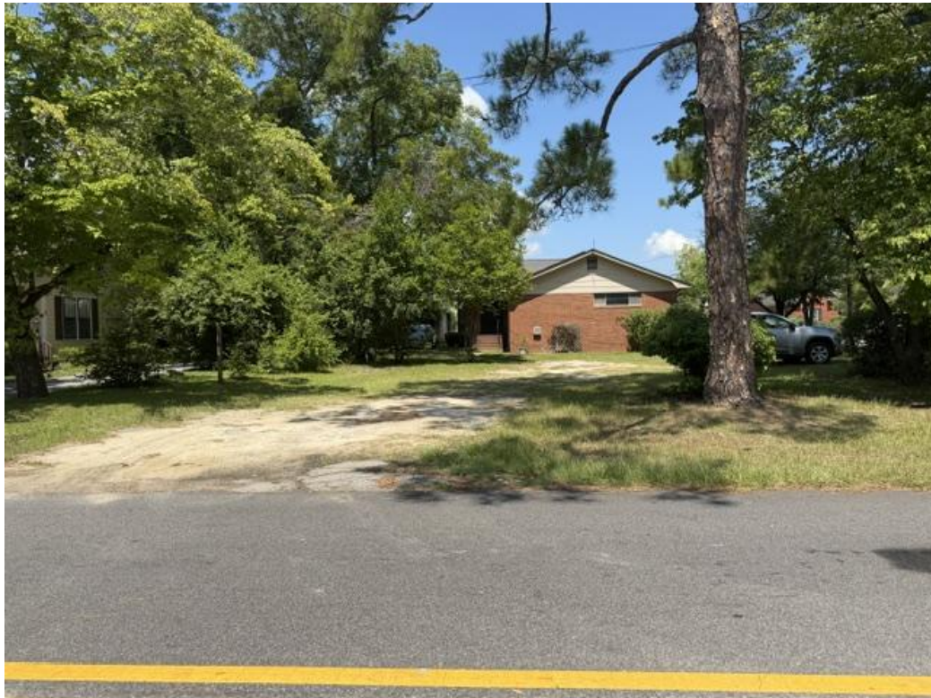
Subject property: view of the east side elevation from the ROW on Donaldson Street, facing west.
